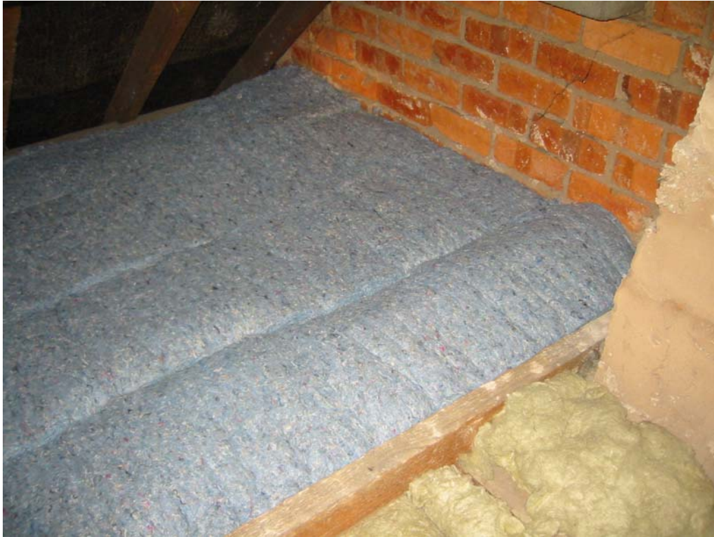
Photo 3. Recovery Insulation laid at right angles to joists above Rockwool.
